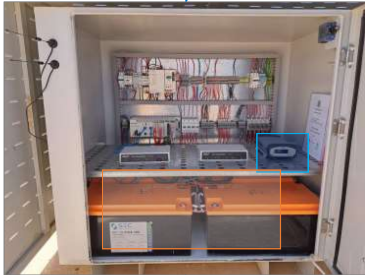
Typical KSACORS Cabinet Component's
