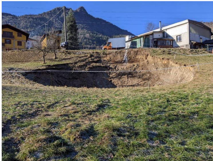
Figure 2: Sinkholes already present in the site
