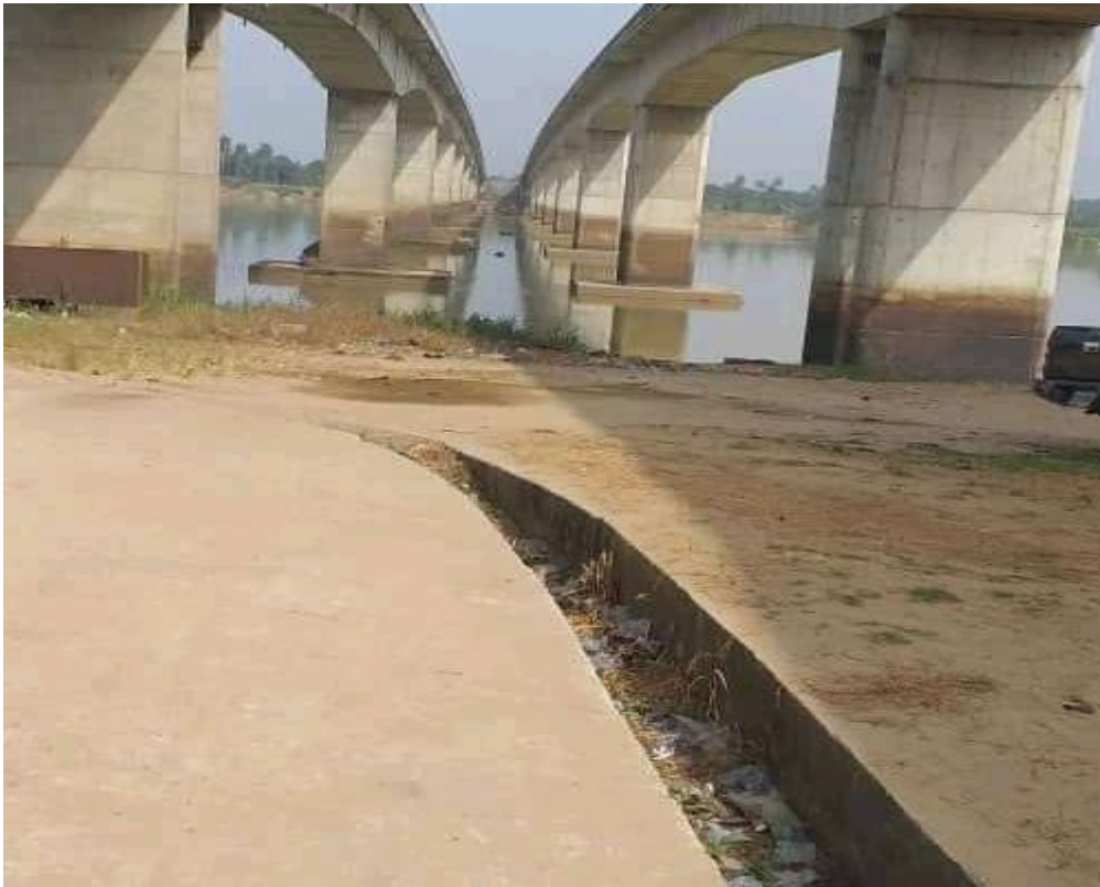
Figure 2: Tidal and Flood Marks on the Legs of Patani Bridge across River Niger Delta. Source: Hydroark Library 2019.
