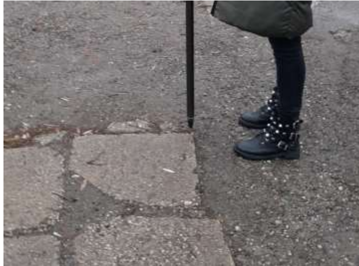
Figure 4: Naturally signalized GCP
