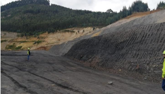
Profile of slopes Mina San Antonio.
