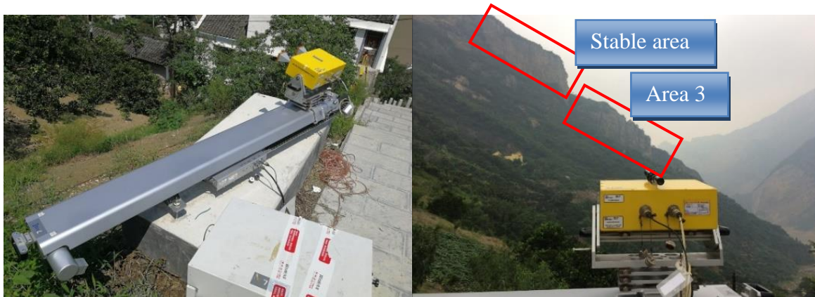
Figure 3: Installation of IBIS (left) and monitoring scene (right)
