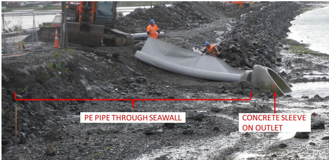
CIPP LINER INSTALL
