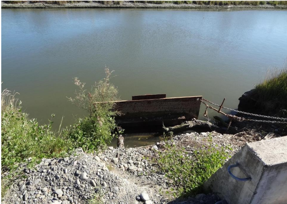
Photograph 2: Steel plate positioned to block a stormwater outlet within the tidal reach of Avon River, New Brighton, to prevent tidal inflow
