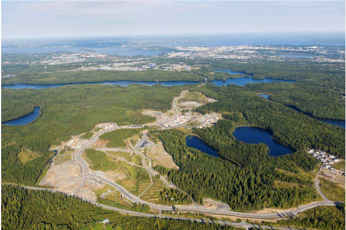
Figure 2: Oblique (2011), 330 dwellings have been constructed
