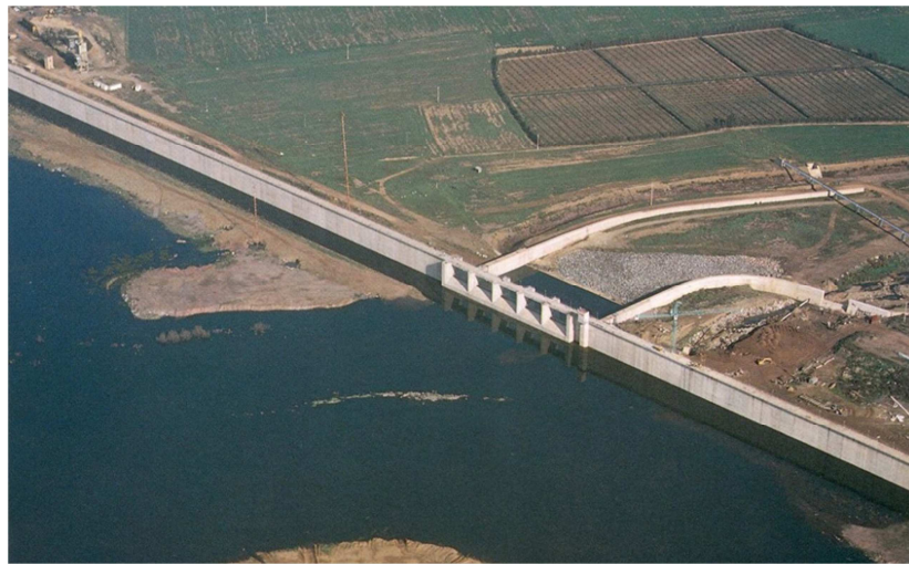
Fig. 1. Aerial view of the Genna Is Abis dam.
