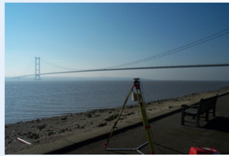
GPS monitoring of the Humber Suspension Bridge
