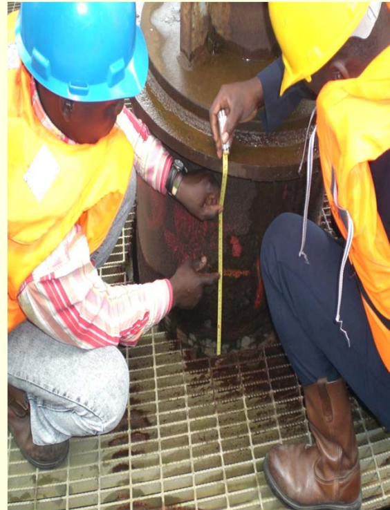
Check on the 1m mark at GB-3 location.
