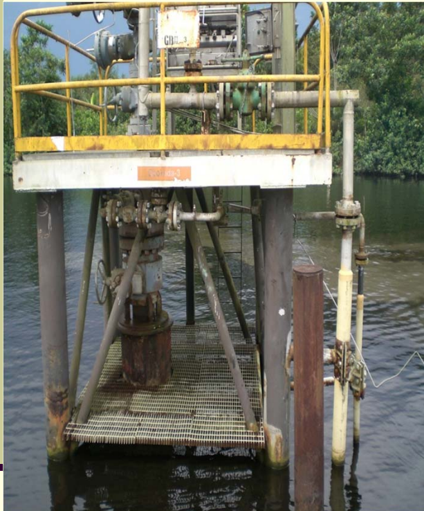
Olero GB-3 location with the 1m mark.
