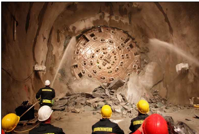
Fig. 2: Cut-through of the TBM on 15 October 2010.
