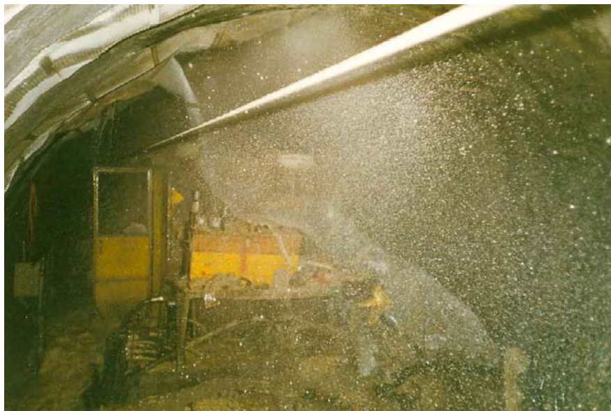
Fig. 10: Blow-out from borehole at 5553 m. A mixture of sugar grained dolomite and water with 1000 m overpressure filled the tunnel. Photo R.Volpers [6]
