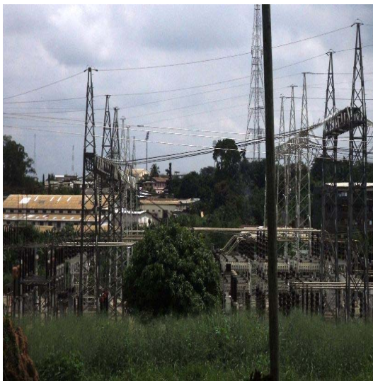
Fig. 7.0 Previous photo of the Substation (left open)
