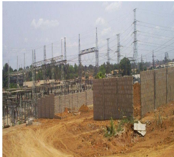
Fig. 8.0 new walls around the station
