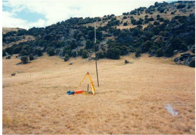
Profile End Point - Concrete Post destroyed by frost
