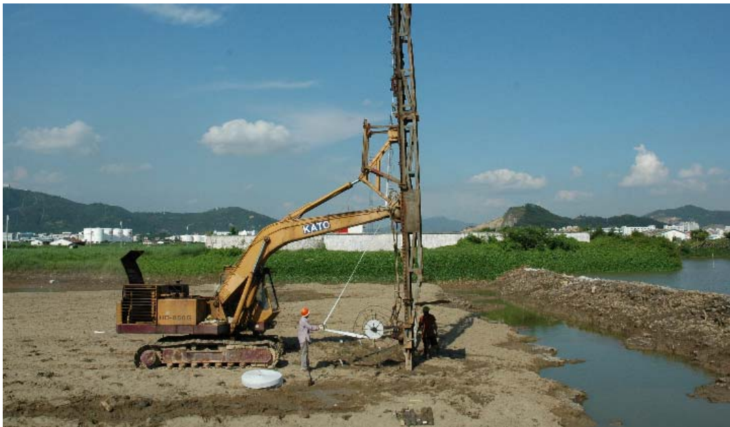
Fig. 2 Installation of Wick Drains
