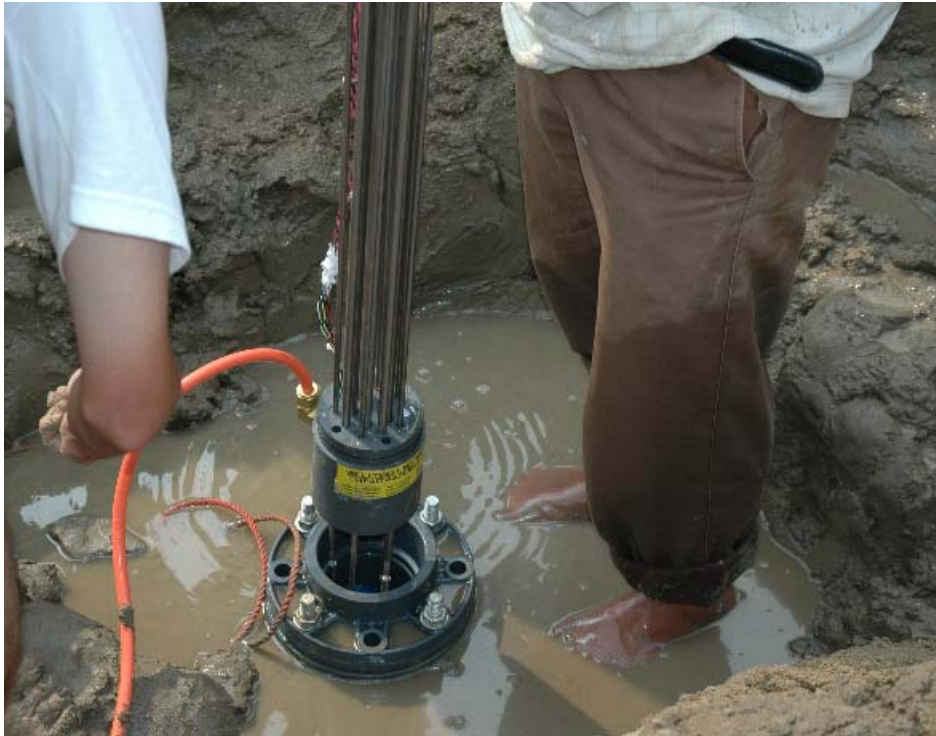
Fig. 3 Installation of Sub-Surface Extensometers
