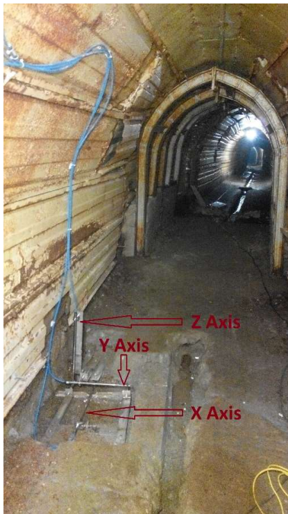
Figure 5. Alexis adit crack meter
