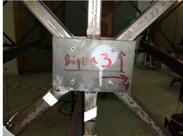
Figure 13: The center joining section of the North side of section 3.
