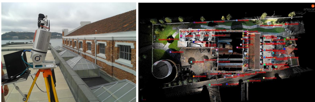
Fig. 3 TLS and photogrammetric survey acquisition (left) and resulting point cloud (right)
