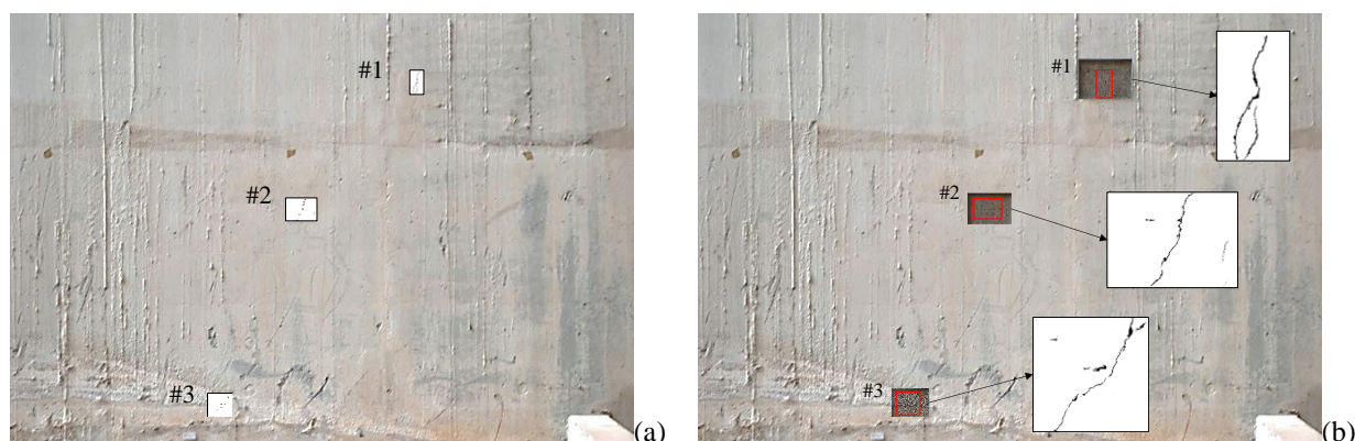
Figure 10. Map of critical cracking areas analysed: (a) location of the areas analysed; (b) zoom of the local areas.
