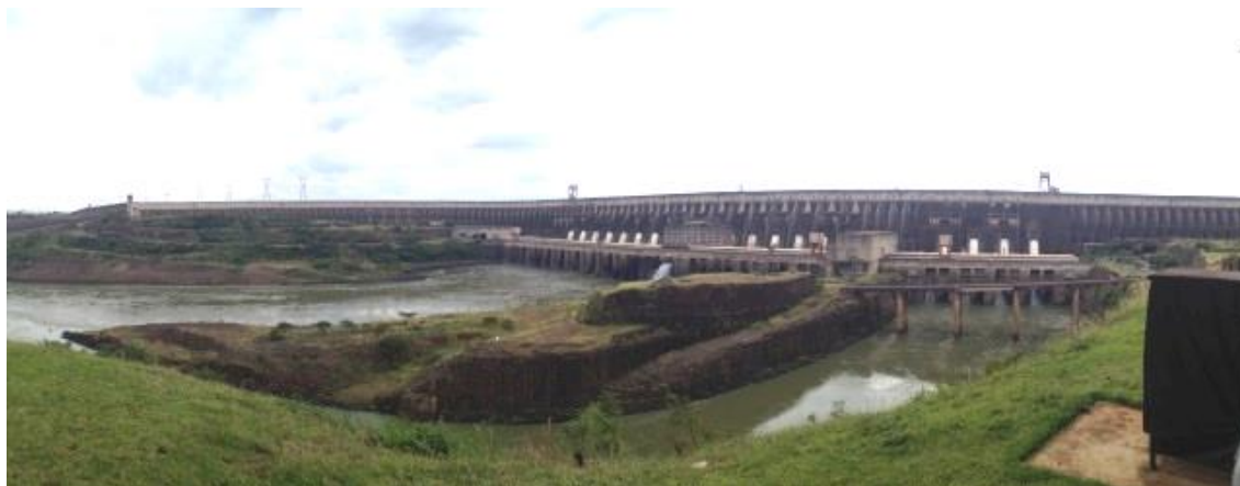
Figure 1. General downstream view of Itaipu dam.
