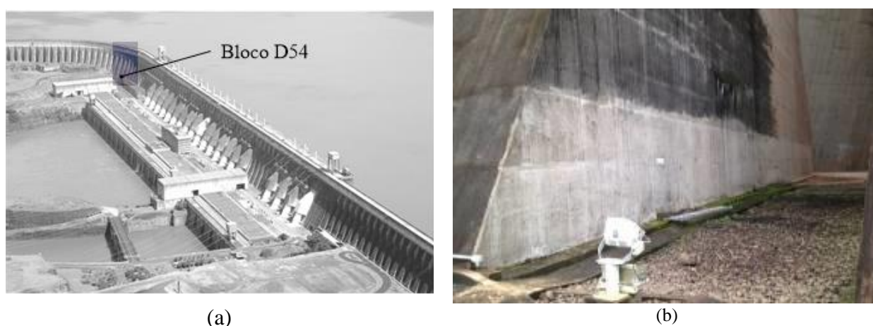
Figure 2. Itaipu dam, block D54: (a) location; (b) surface to assess.
