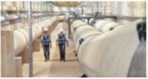
Common Services Tunnel This tunnel system houses power cables, Pipes and other infrastructure for the Marina Bay area
