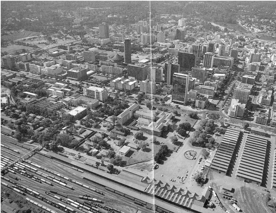
Photograph 2: Part of Nairobi City Centre showing different tower blocks with offices on the same land parcel.
